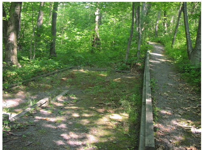
Trail Section 12 along existing path.
