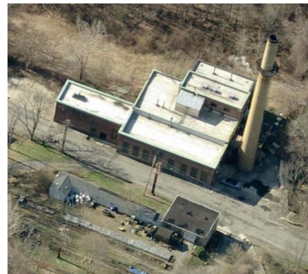
Power Plant Power Plant
